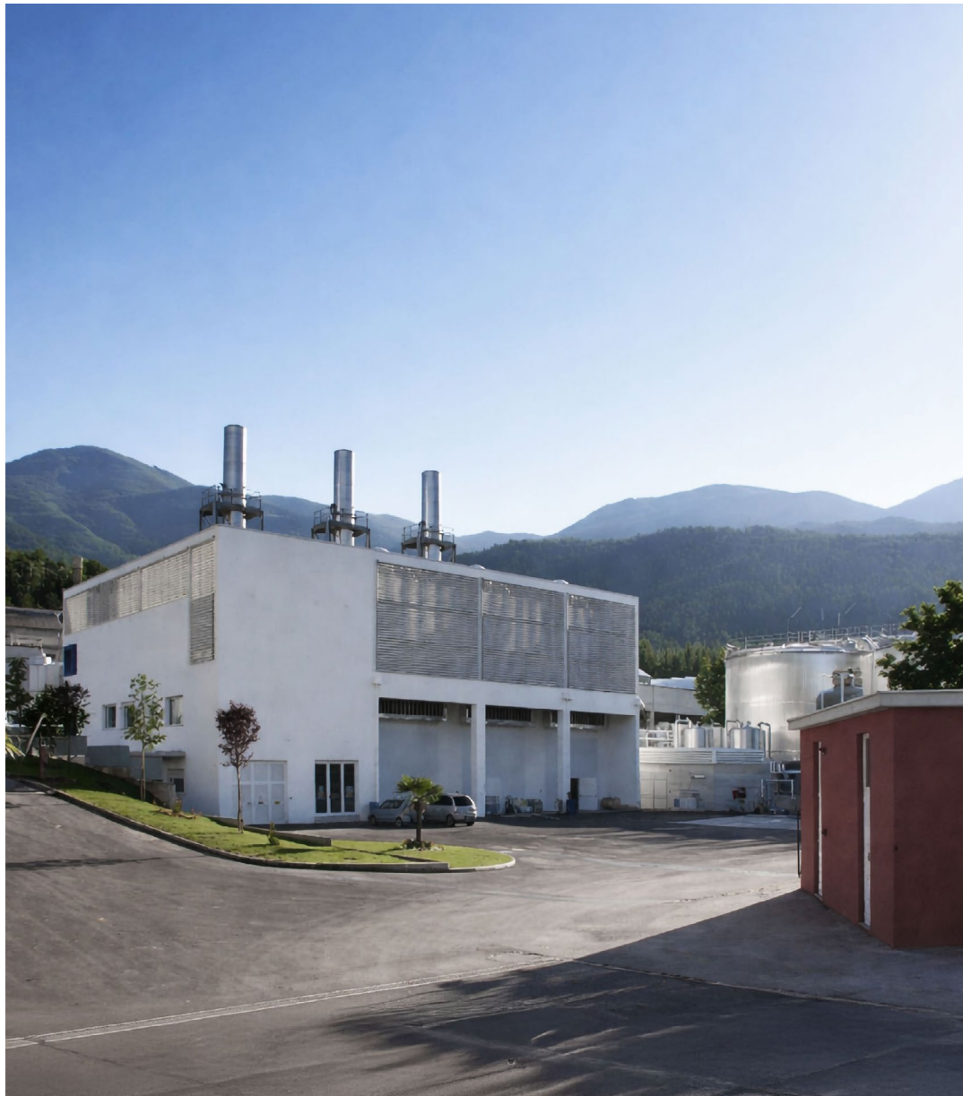
Electric power generation plant fueled by bioliquids. BEG, Guarcino (FR)
